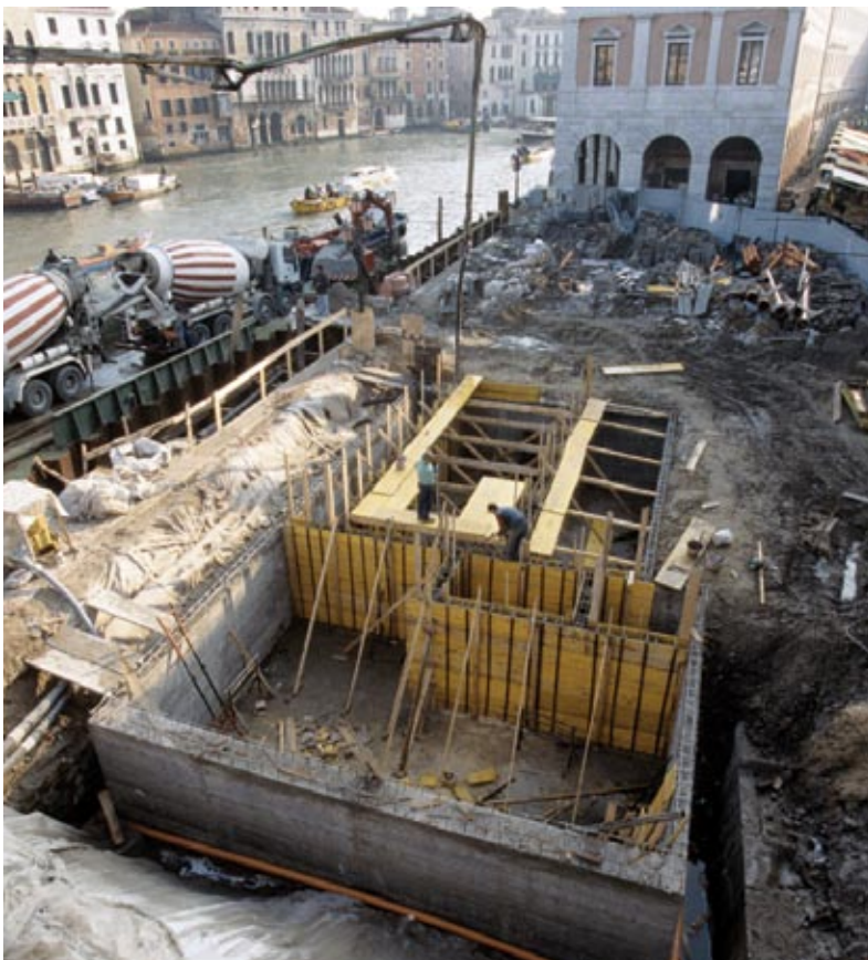
Rialto, the new water purification plant in Campo della Pescheria.
